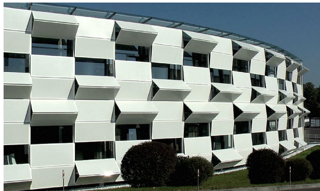
Figures: 2.95 Musical envelope as wave contour (3D Spectrogram in SignalScope Pro); 2.96 Musical scoring as surface reticulation; 2.97 Sculptural profile (Anton Smit, Oblivion of the Waves , date unknown); 2.98 Architectural facets (Howard Engine Company No. 34 firehouse, 1864, converted to a private residence in 2009); 2.99: Architectural features (Kiefer Technic Showroom, circa 2007)
